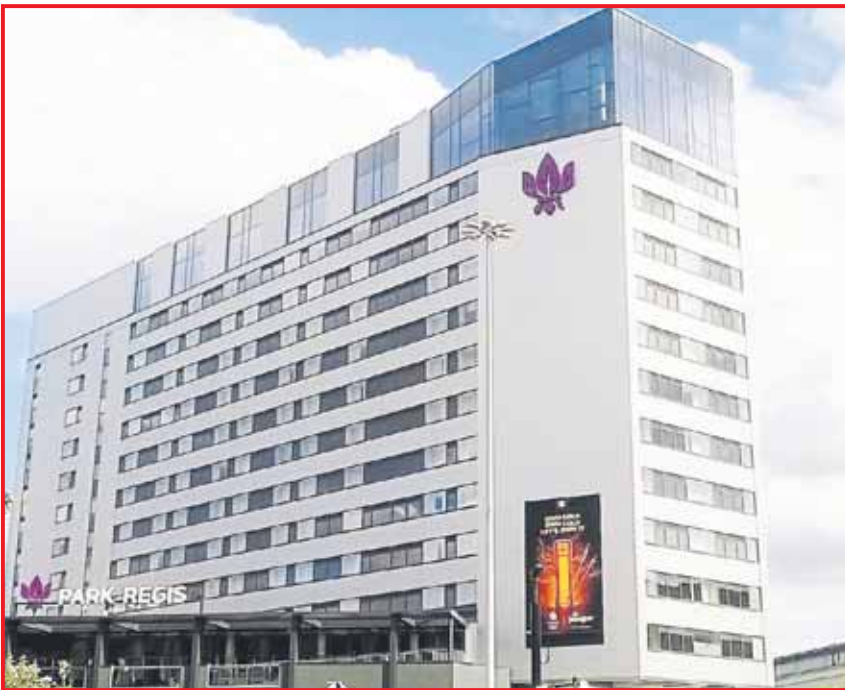
Among a string of landmark projects across Birmingham, APiC worked on the new Park Regis Hotel
